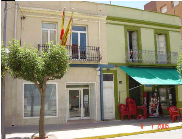
Accessos no adequats
